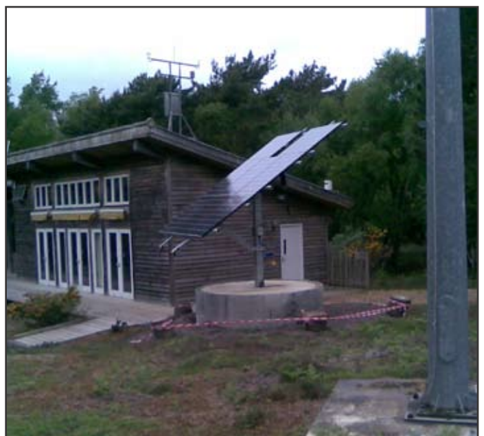
Figure 7: Studland Study Centre with solar panels
